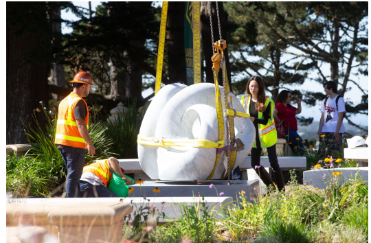
On site during installation — University of San Francisco
