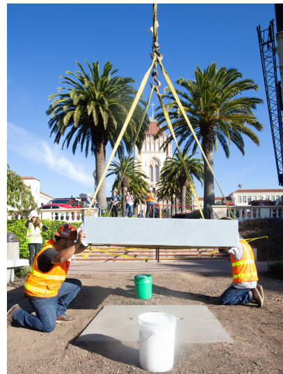
Base installation over the engineered footing
