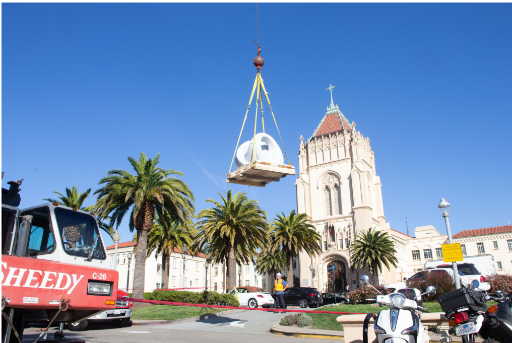
Crane-assisted installation — Lone Mountain campus | Photography: Natalie Schrik
