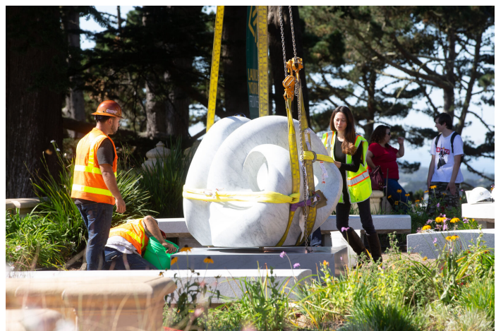
On site with the rigging crew
