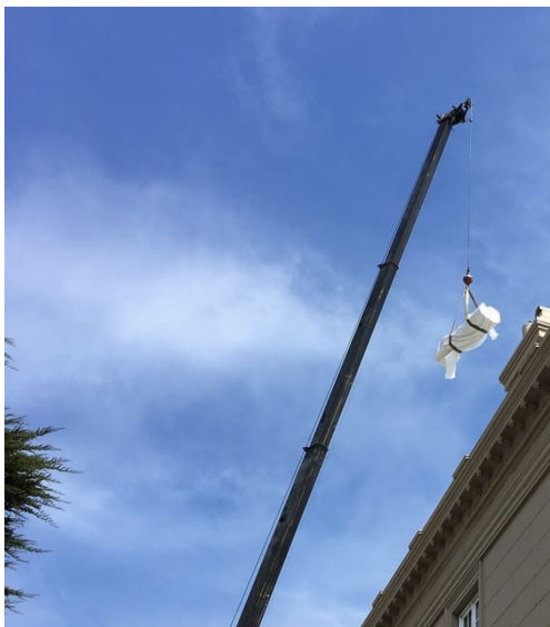
Crane installation — Le Petit Trianon garden
